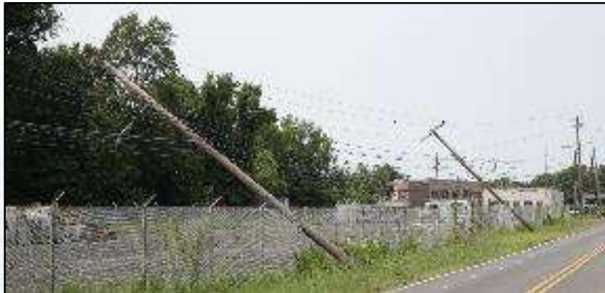
Unplanned Storm Damage Electrical Repair
